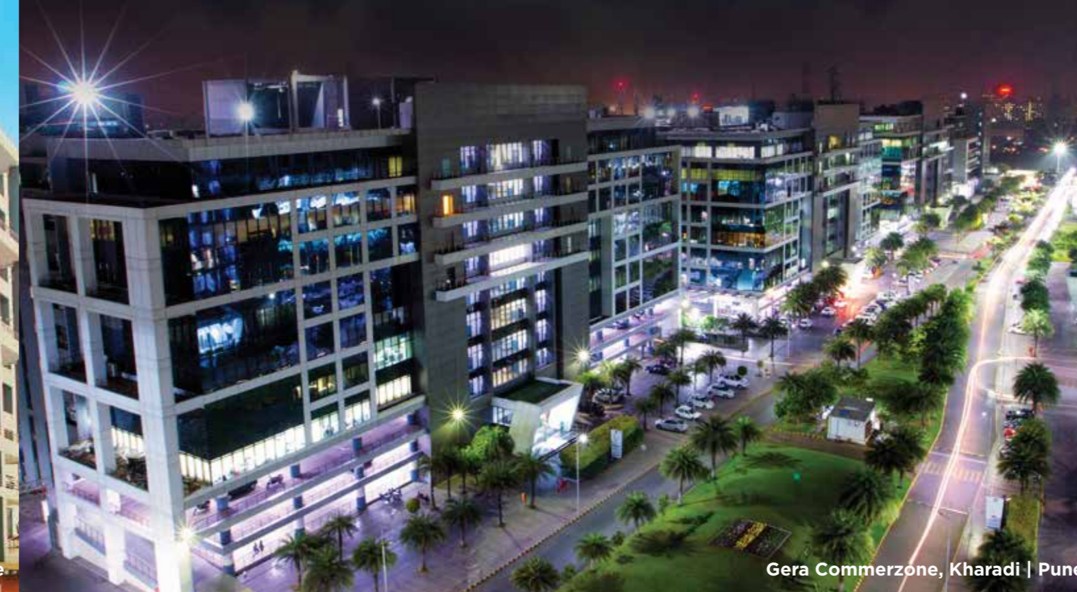
Commerzone, Yerwada | Pune
